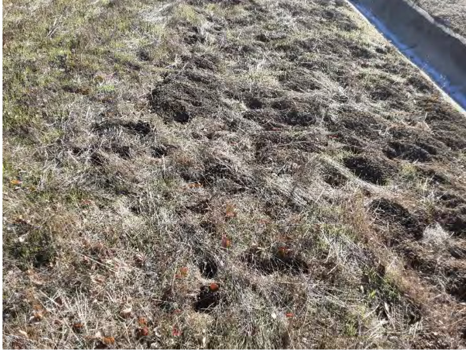
Photo 1. View of rodent burrows on the previously graded slope on the eastern side of Magee Ranch Road.
