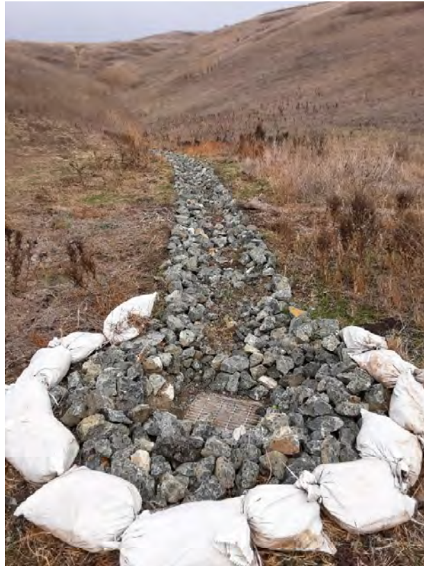
Photo 15. View of erosion repair with drain rock and new direct inlet on Sunhaven Trail.
