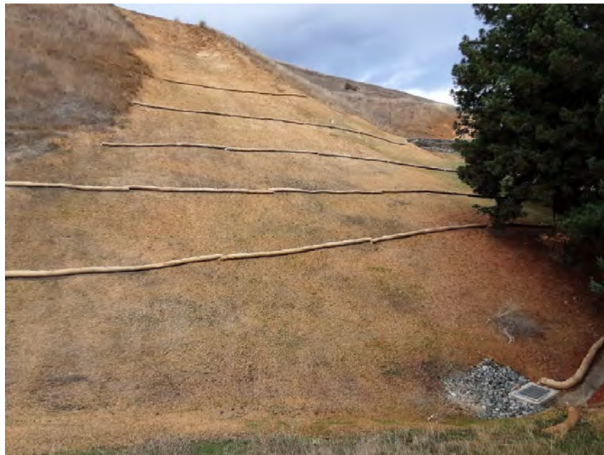
Photo 14. Repaired slope with hydroseed and drain rock behind 158 Sunhaven Road.
