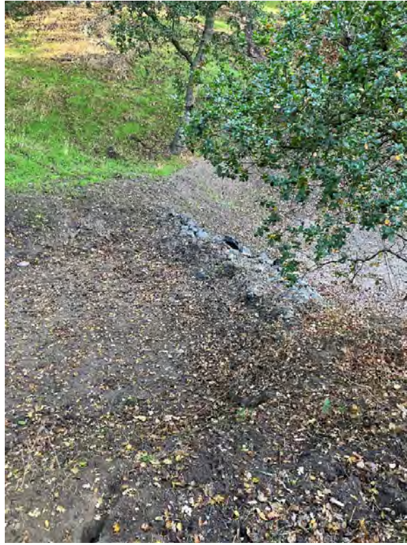
Photo 13. View of basin behind 138 Windover Drive at capacity.
