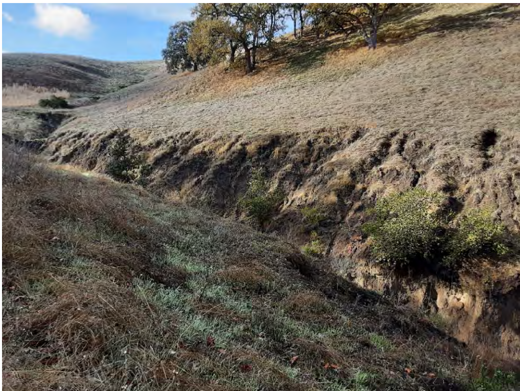
Photo 10. View of significant erosion in the ravine south of 138 Windover Drive.
