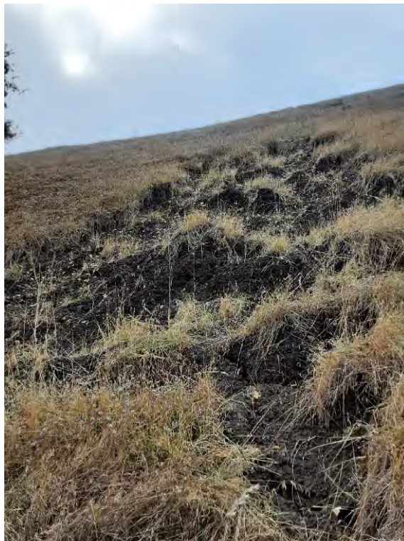
Photo 4. View of recently active landslide above repair behind 15 Brightwood Circle.
