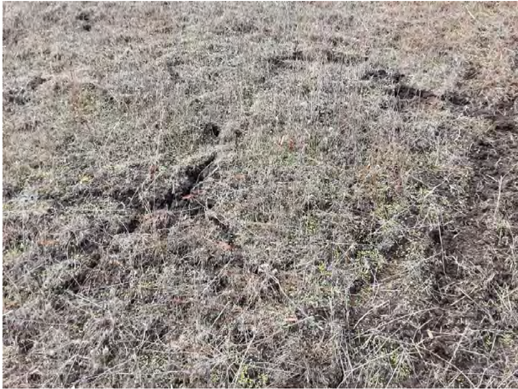
Photo 7. Soil cracks and creep observed behind 19 Maplewood Drive.
