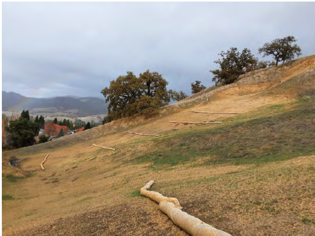
Photo 16. View of repair with new cleanouts and rockwall behind 116 Shadewell Drive.
